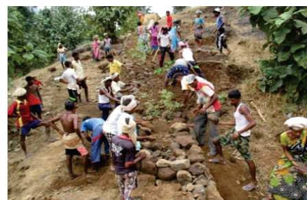
Cattle protection trenches
